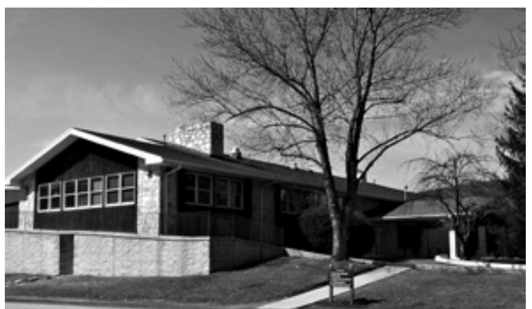
The first phase of a $20 million upgrade to Ski Liberty facilities will begin with the demolition of the existing Club House building.
