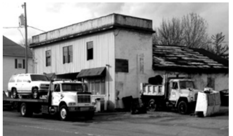
If plans are approved, the dilapidated East End Garage on East Main St. will be torn down and replaced by a Dollar General store.
