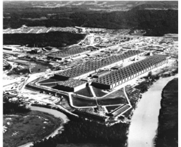
K-25 at Oak Ridge served as the United States' principle gaseous diffusion facility for the enrichment of uranium for use in nuclear weapons. At one time, it was the largest building in the world.
