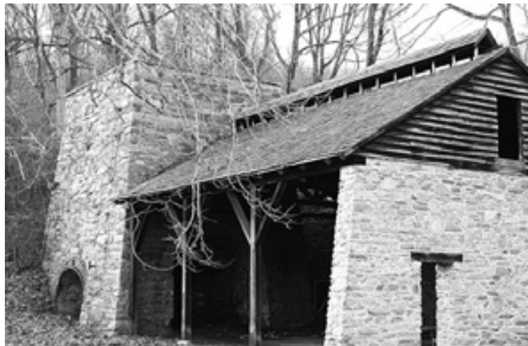
Catoctin Furnace - A cemetery for the slaves working at the furnace was disturbed in this area when Rt. 15 was expanded from 2 lanes to 4 lanes.
