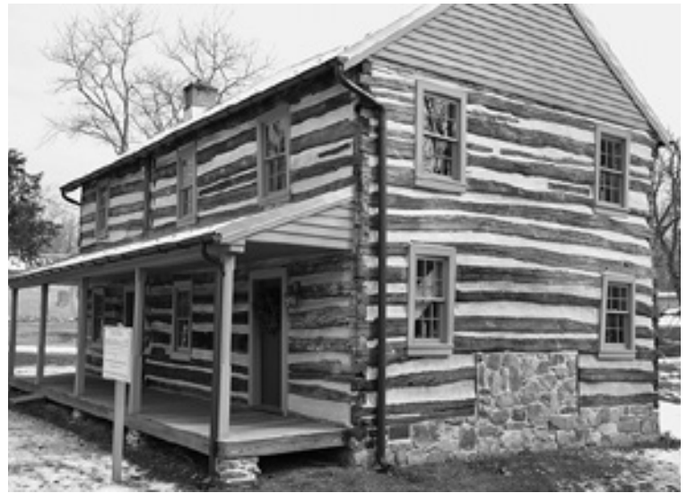
Collier's House - On Catoctin Furnace Rd. just south of the iron furnace
